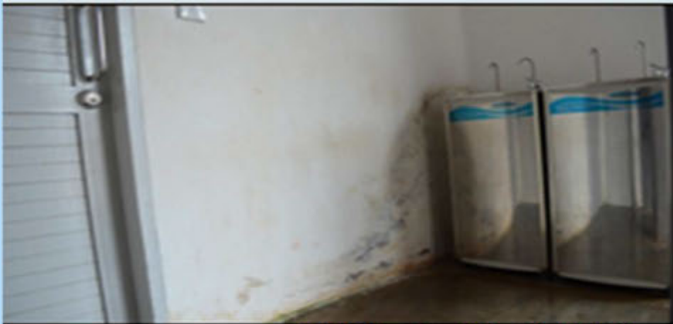
SMKA Sheikh Haji Othman Abdul Wahab, Kuching, Sarawak - Kesan Resapan Di Dinding Tandas Guru Blok Akademik (05.03.2015)
