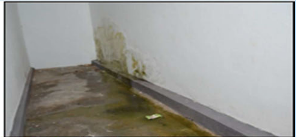
SMKA Sheikh Haji Othman Abdul Wahab, Kuching, Sarawak - Kesan Resapan Di Dinding Tandas Guru Blok Akademik (05.03.2015)
